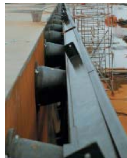
▲ Canal Bridge Barrier (GERMANY)
