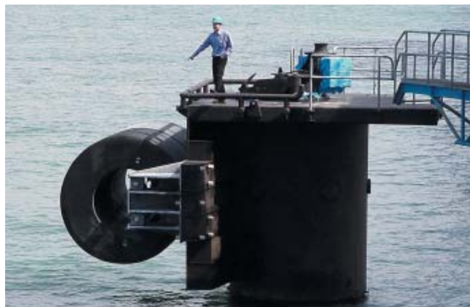
▲ Power Station Coal Berth
