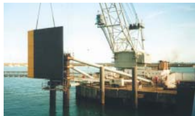
▲ During installation of Dunlaoghaire HSS Berth (IRELAND)
