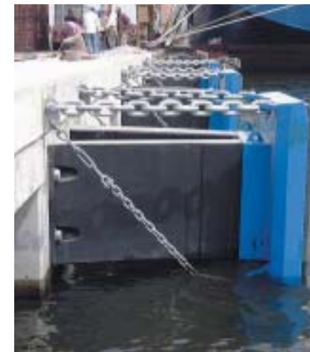
▲ Port Said Container Terminal (EGYPT)
