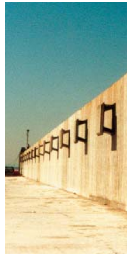
▲ Hydrolift Dry Dock, Setubal (PORTUGAL)
