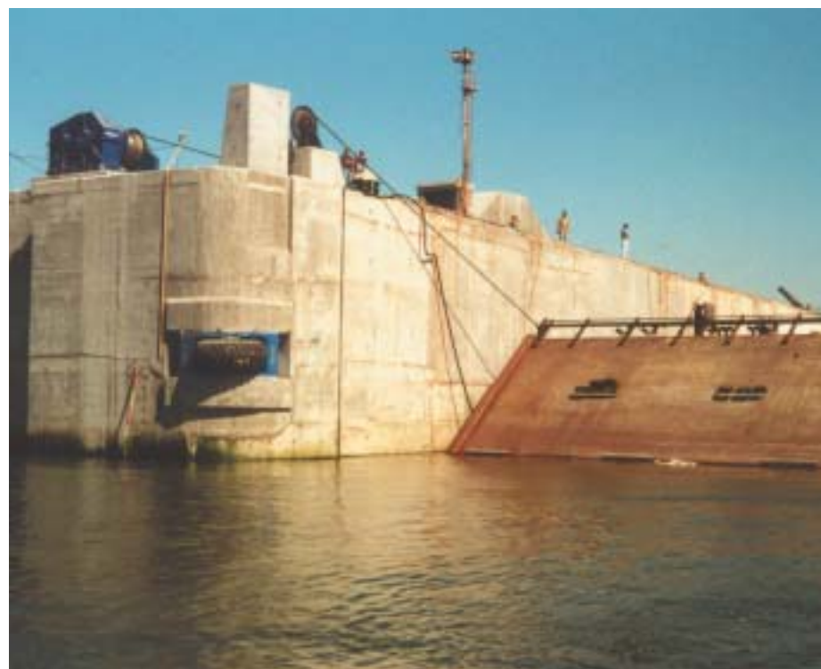
▲ Lisnave Hydrolift Facility, Setubal (PORTUGAL)
