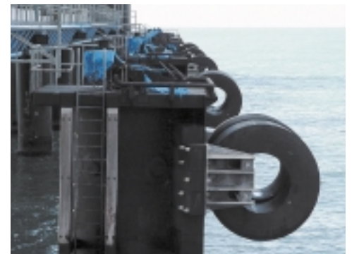
▲ Coal Terminal Dolphins
