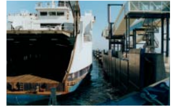
▲ Mukran Fender Wall, Sassnitz (GERMANY)
