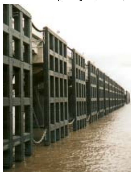
▼ West Lead-In Jetty, Immingham (ENGLAND)
